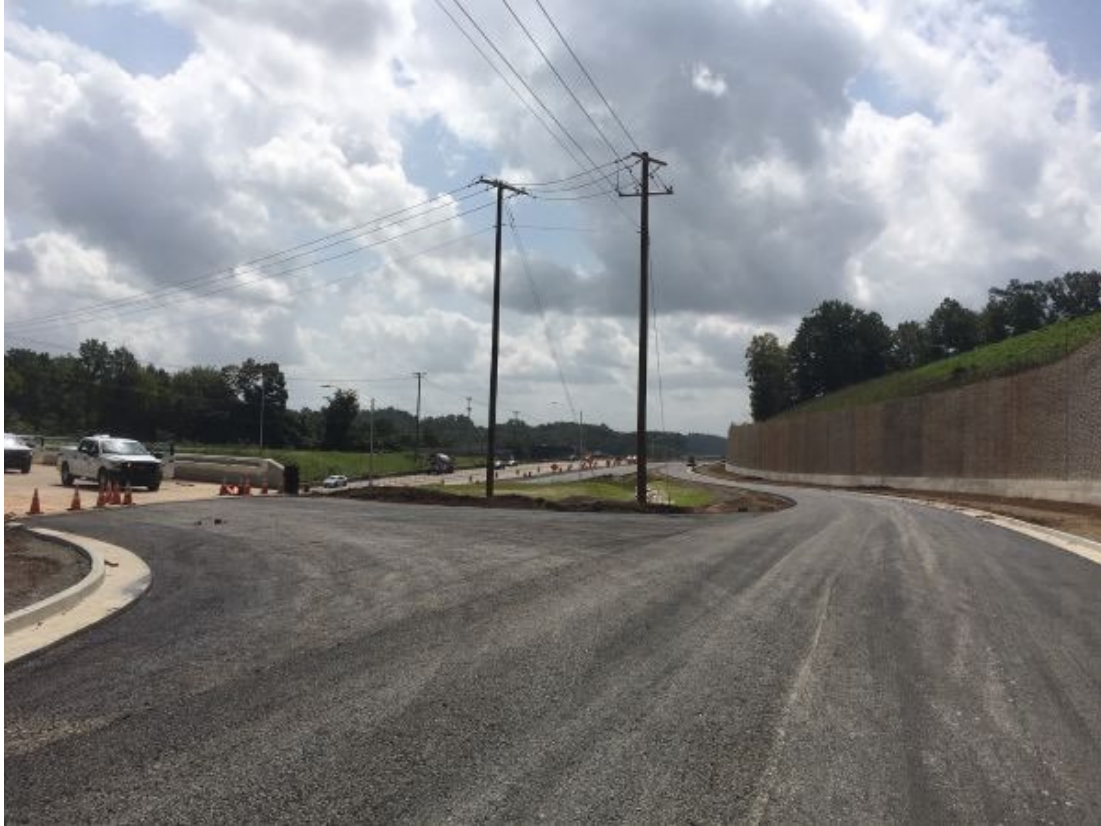
Alcoa Highway Construction, September 2020
