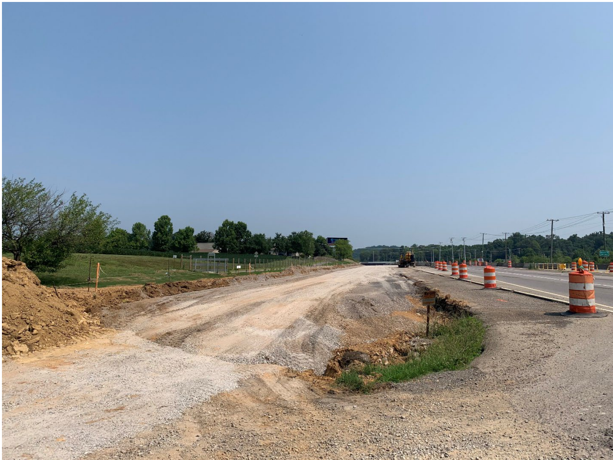
Alcoa Highway construction, July 2021
